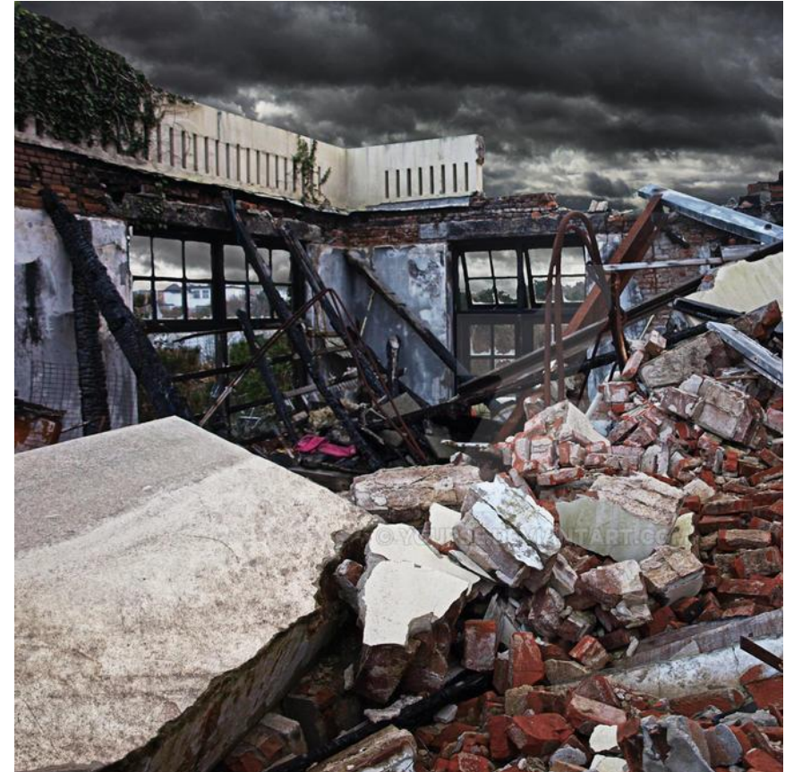
Fig. 3.1 Destruction caused due to earthquake
